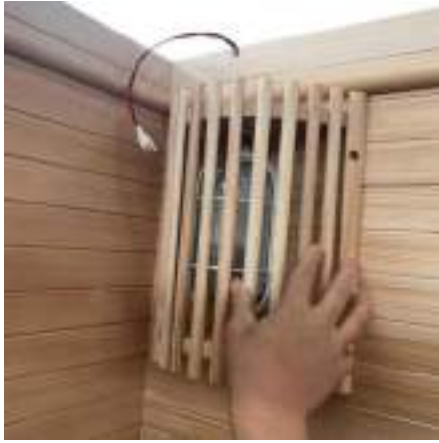
(17) Assemble wood cover for sauna lights 3x25 mm 8 pcs
