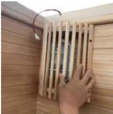
(15) Assemble wood cover for sauna lights 3x25 mm 8 pcs
